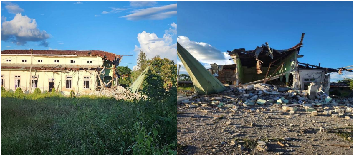
Tanang U Koi church damaged by airstrike
